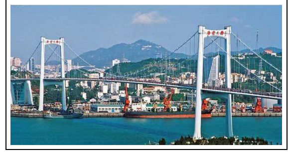
Figure 2. Xiamen Haicang Bridge.
